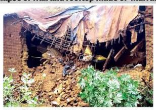
the walls became wet and collapsed, bringing down the rooftop as well. The most surprising thing here is that nobody heard the noise from falling of the wall.
